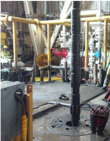
Removing the Intercept® bridge plug nine months after installation
