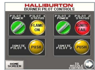
HMI Display screen for ignition and pilot flame detection
