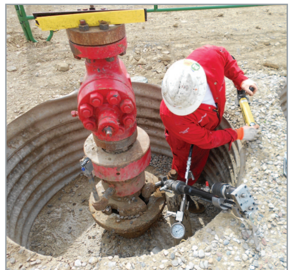
Compact hot tap units enable easy access in confined spaces.
