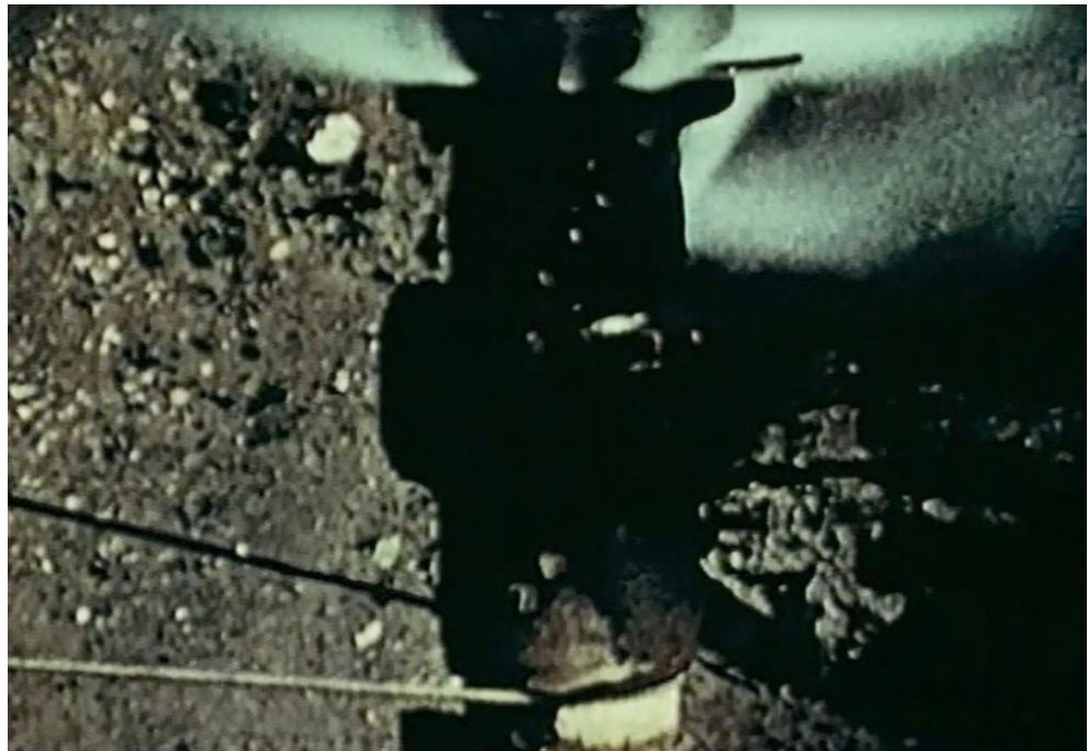
Figure 5. A sandline cutter removes the wellhead to allow for the well to be capped on the clean, smooth casing.
