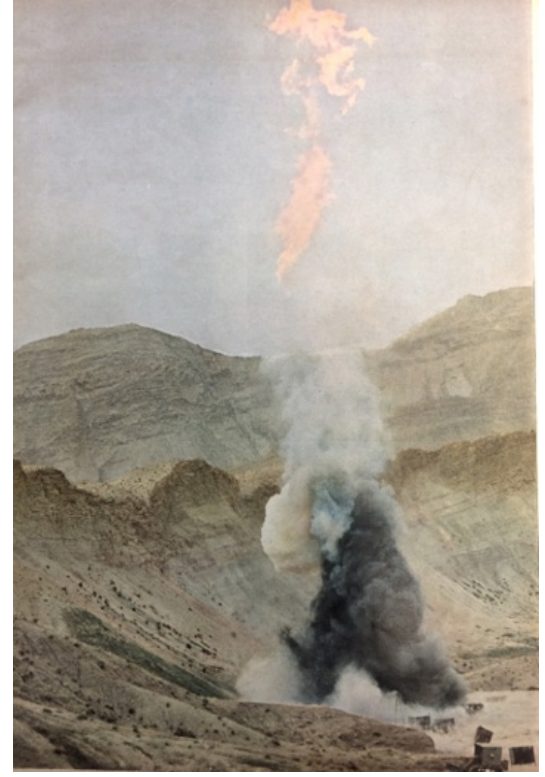
Figure 4. Blowout fire being snuffed out by 1,100 pounds of explosives. Courtesy of R. Hatteberg and LIFE Magazine.
