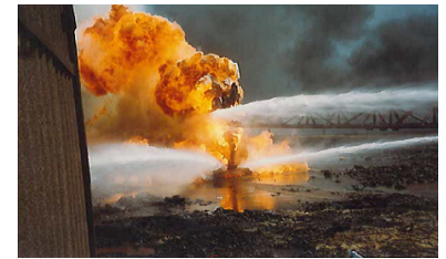
Figure 2. Boots & Coots well control experts spray water to cool a wellhead and potentially extinguish the fire. (Photo courtesy of R. Hatteberg)
