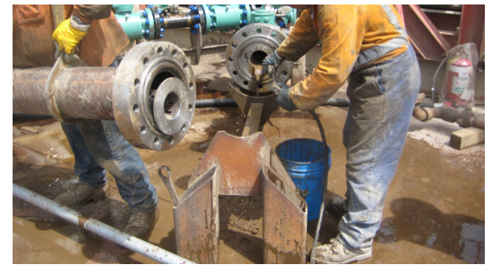
Rock catchers collect large amounts of cuttings
