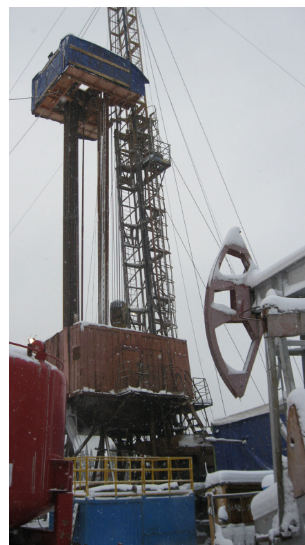
Rig for Bashneft Sukhoyazskoye Well 5
