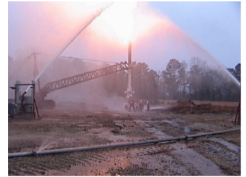
The blowout well is capped, and a Venturi tube and diverter system are in place.
