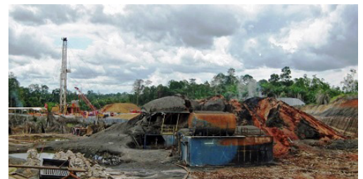
Figure 3. The relief well can be seen in the left background, 500 feet (152 meters) behind the destroyed target well.
